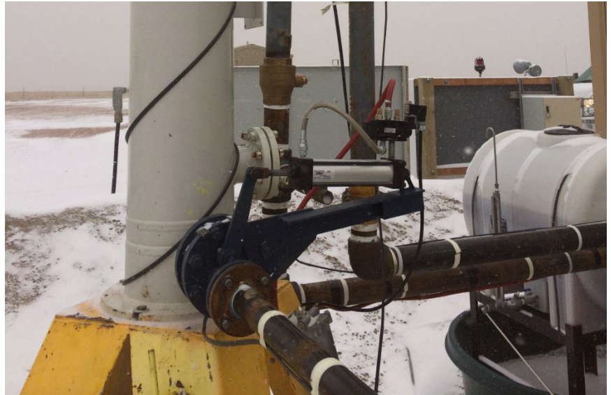
Produced Water De-sanding Hydro-cyclone, Ambient Temp, 100psi
